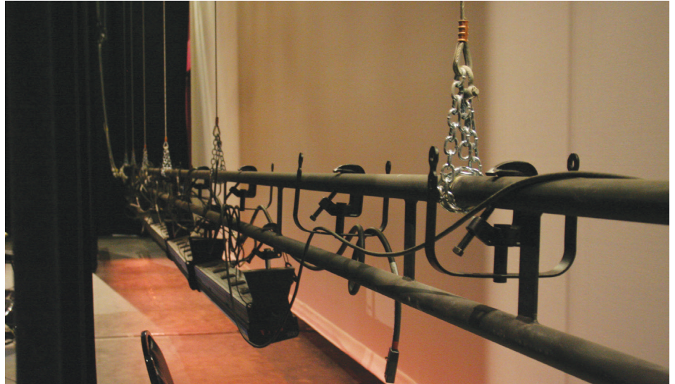
A lighting pipe with cable hooks. No tie line necessary!
